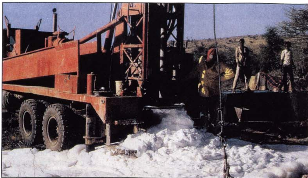
Using foam with air rotary to drill and clean out a well located near the Somali/Ethiopian border.
